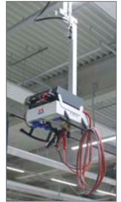
E-BOX with ELTEK charging computer
